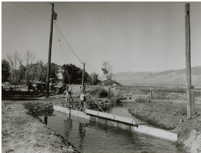
Above left: location of irrigation diversions on the Lemhi River; above right: perforated fish screen operated by waterpower on canal in the Lemhi Valley; lower left: perforated fish screen operated by electrical power in the Lemhi River. Photos and diagram, circa 1957. Source: Lemhi County Historical Society in the Gebhards Collections. “The Effects of Irrigation on the Natural Production of Chinook Salmon in the Lemhi River” by Stacy Gebhards. A thesis submitted in partial fulfillment of the requirements for the degree of Master of Science in Fisheries Management. Utah State University, 1959.
