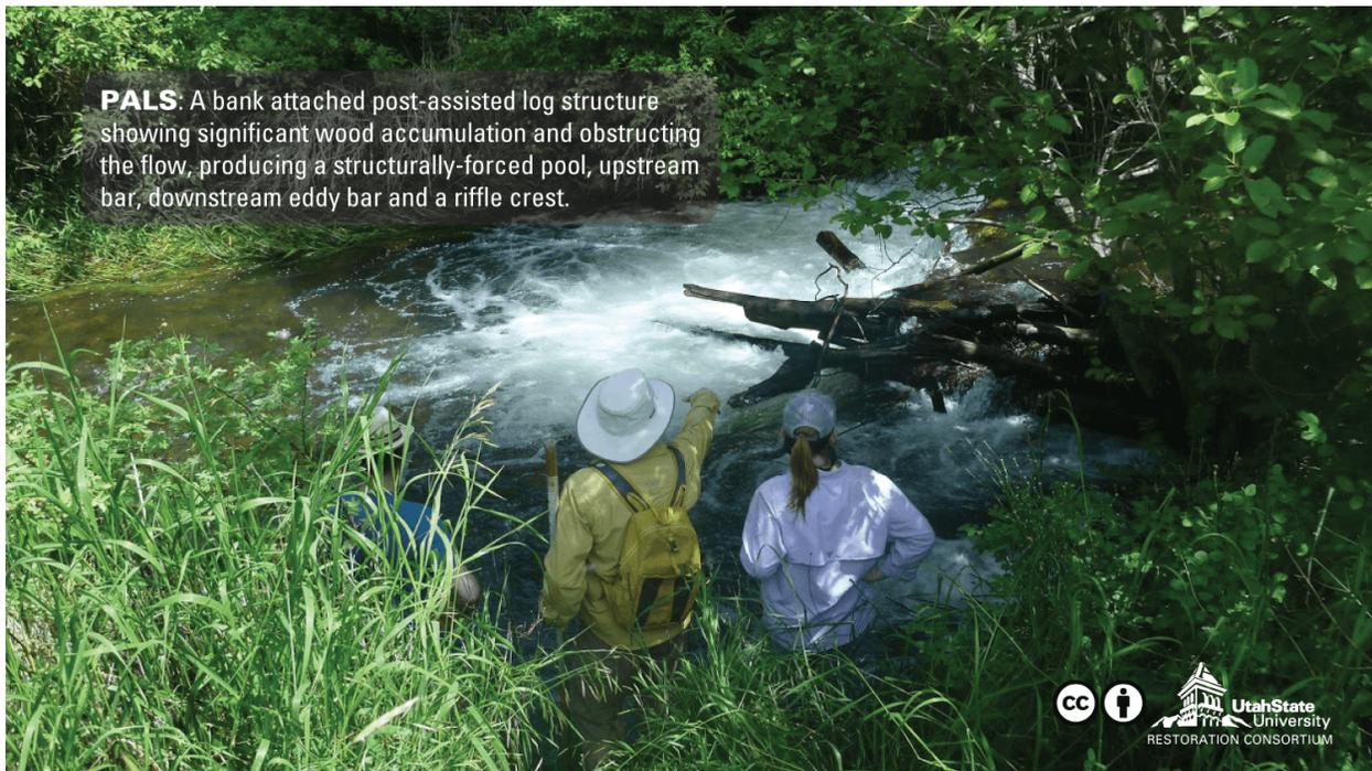
Figure 3 – A post-assisted log structure (PALS) so buried in wood accumulation and sediment, it is hard to recognize.
