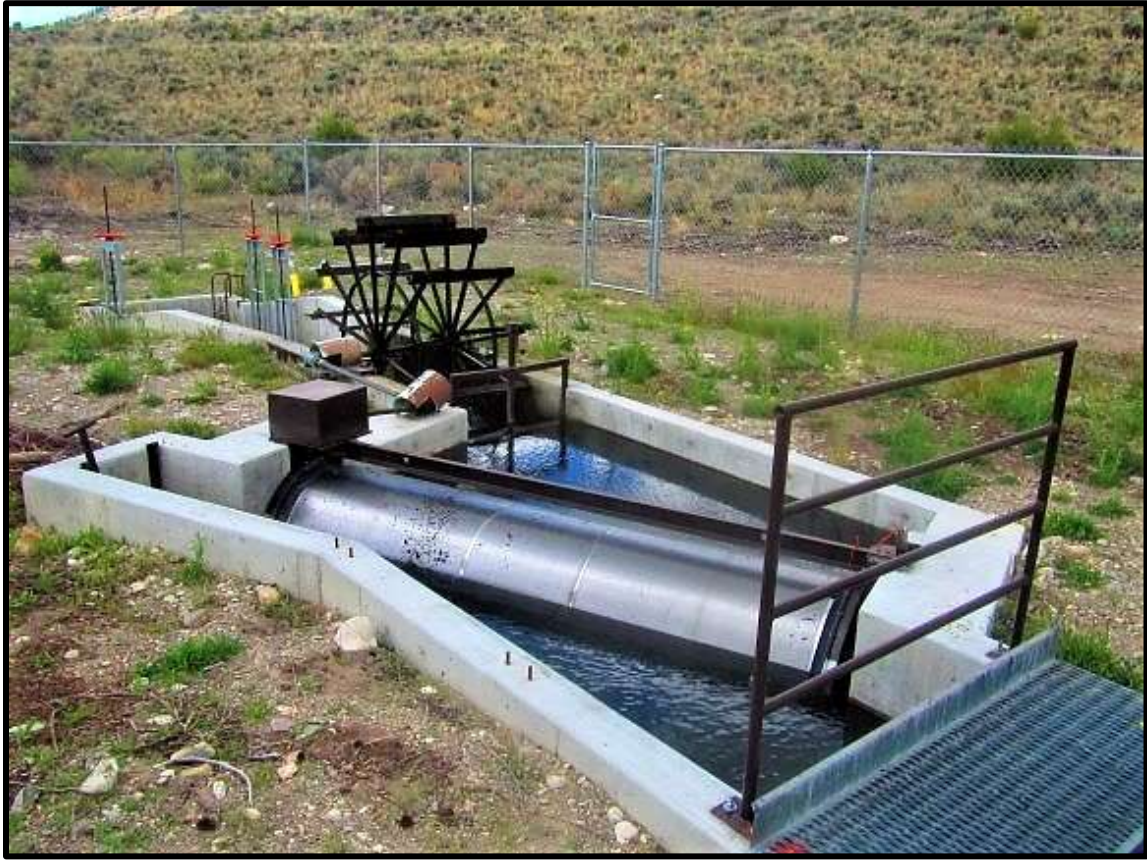
Photo 2. New NMFS criteria fish screen installed at the Hawley Creek-02 (LHaw-02) diversion in 2017.
