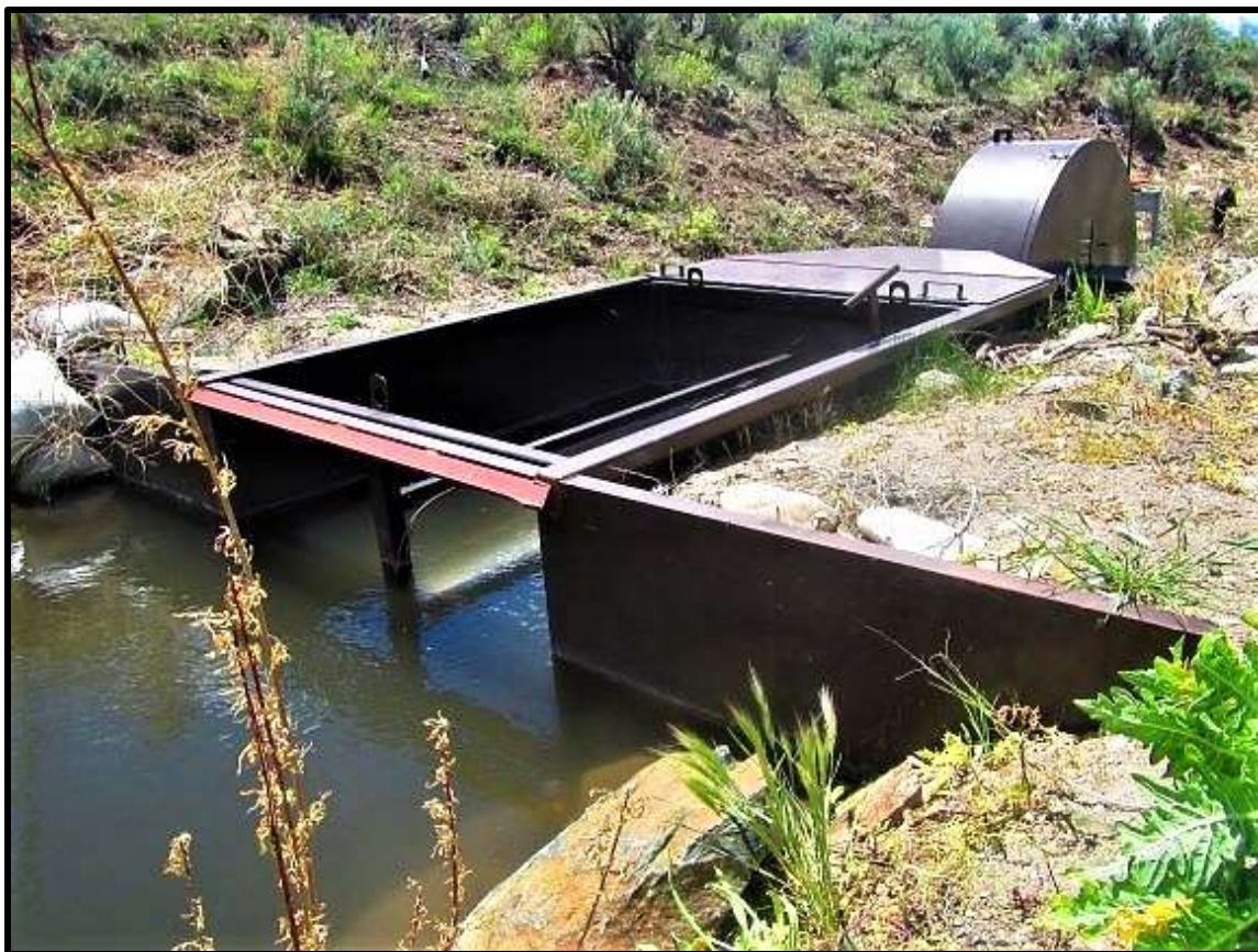
Photo 3. New NMFS criteria closed drum fish screen installed at the Canyon Creek (LCC-03) diversion in 2017.
