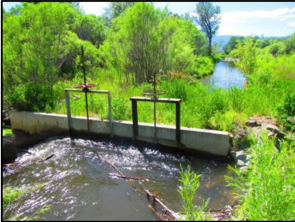
Photo 15. The L-08A ditch was enlarged to accommodate the additional water.
