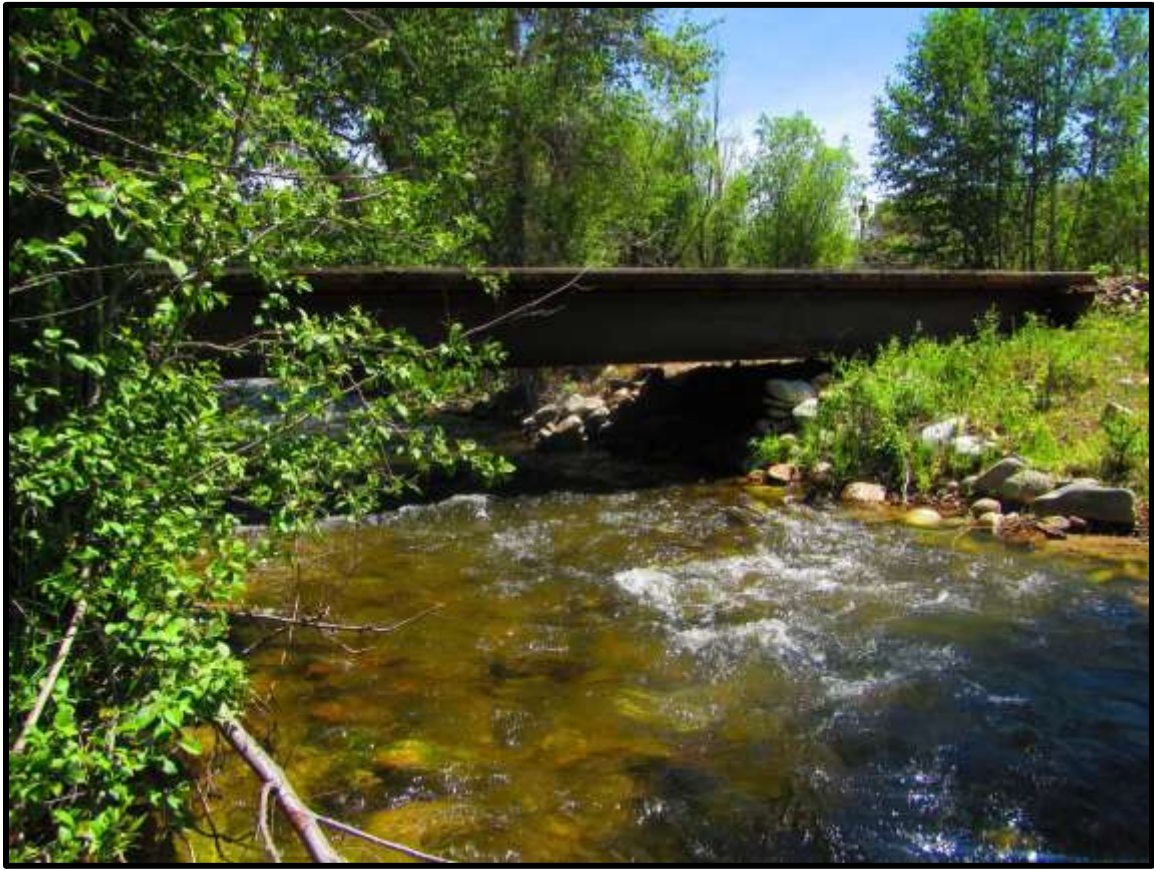
Photo 7. The old Carmen Creek -03 (SCC-03) access bridge was replaced with a new bridge in January 2018.
