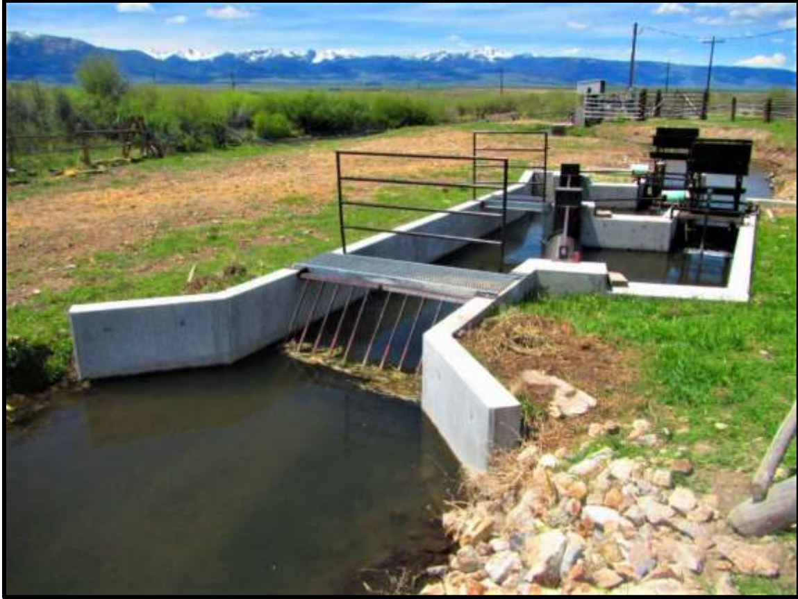
Photo 5. An old fish screen was replaced with a new screen at Lemhi River-62 (L-62) in the fall of 2017.
