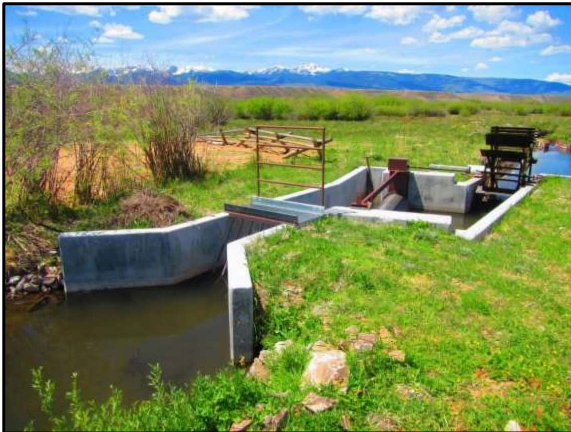
Photo 4. An old fish screen was replaced with a new screen at the Lemhi River-60 (L-60) in fall of 2017.
