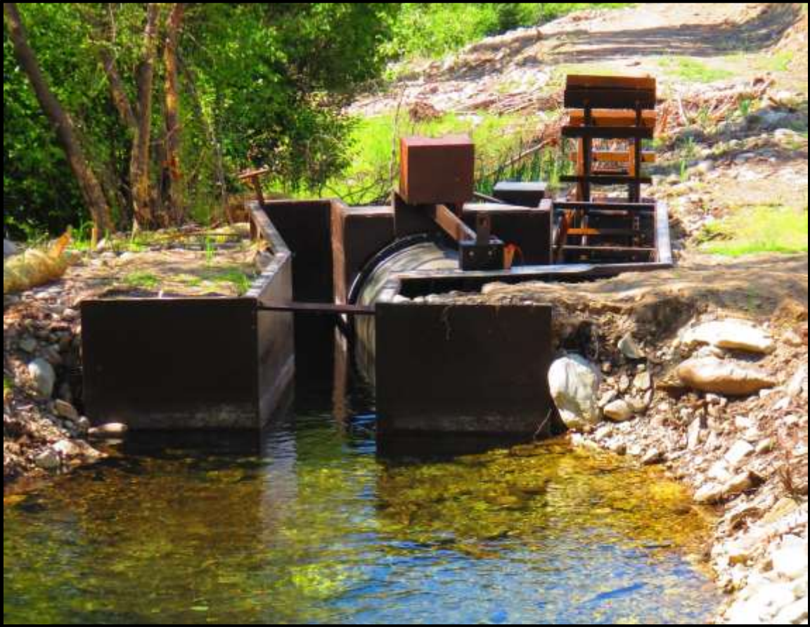
Photo 11. Pratt Creek-02 (LPrC-02) fish screen was installed in spring of 2019.
