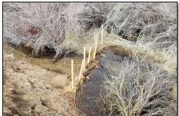
Recently installed BDA; Hulls Gulch, ID
