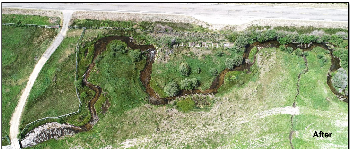
Big Springs Creek, ID; 1 year after construction; Reduced channel width, increased sinuosity, improved shade, and hydraulic diversity using a variety of bank fill treatments (FESL, brush mat, willow clumps, post-line willow-weave, gravel placement)
