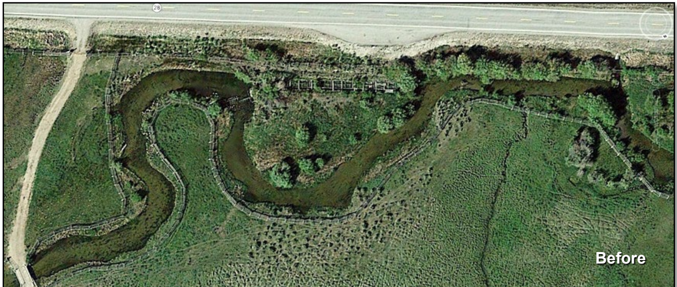
Big Springs Creek, ID; Before construction; Over-widened channel with plane-bed and poor habitat diversity
