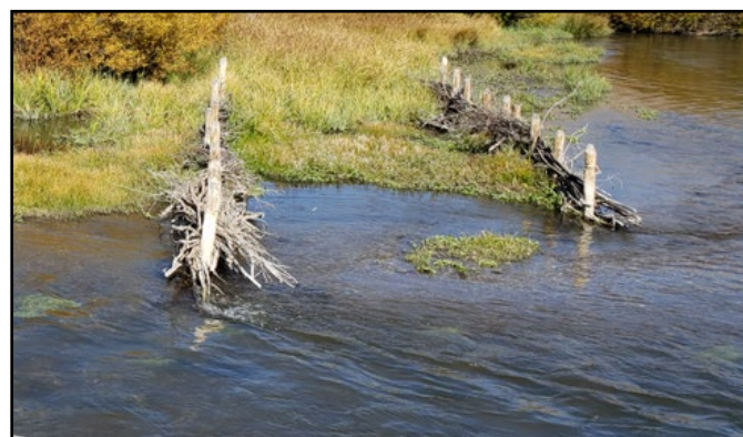
Series of post-line willow-weave bank deflectors creating a point bar; Lemhi River, ID
