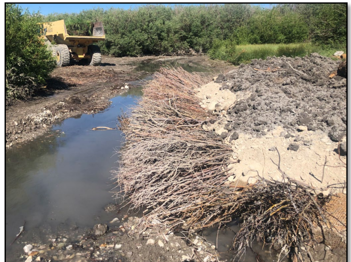
Willow brush layer during construction (Above) and immediately after construction (Below); Lemhi River, ID
