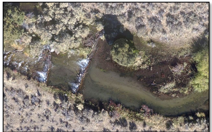
BDA series capturing sediment and raising the water surface immediately after construction; Hawley Creek, ID
