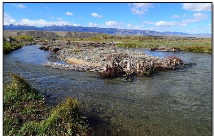
Apex jam constructed of willow clumps; Lemhi River, ID
