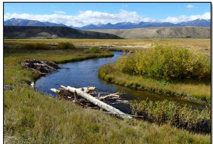
Small and large wood material bank structures immediately after construction; Big Springs Creek, ID
