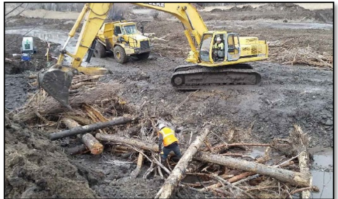
Bank roughening structure during construction; Lemhi River, ID
