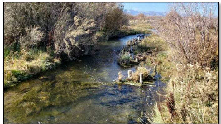
Small wood material structures 1 year after construction; Big Springs Creek, ID
