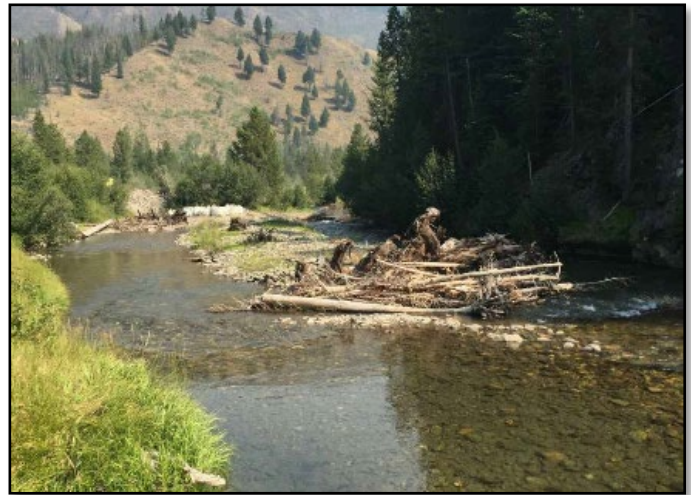
Apex log jam 1 year after construction; Yankee Fork of the Salmon River, ID
