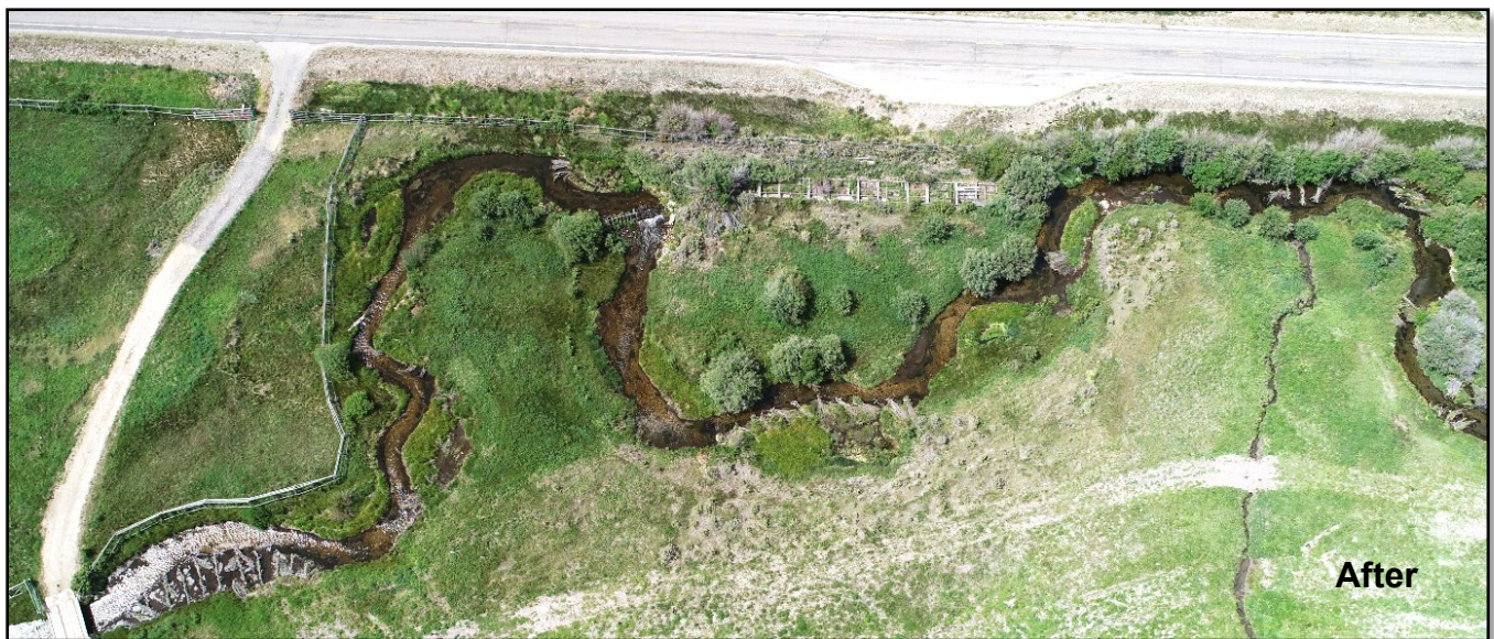
Big Springs Creek, ID; 1 year after construction; Reduced channel width, increased sinuosity, improved shade, and hydraulic diversity using a variety of bank fill treatments (FESL, brush mat, willow clumps, post-line willow-weave, gravel placement)
