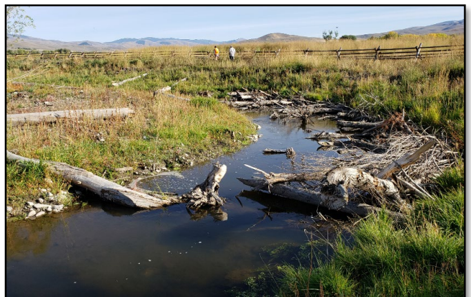
Bank roughening structure on newly created side channel 1 year after construction; Lemhi River, ID
