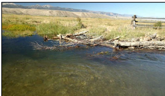
Small wood material bank structures with excavated scour pool immediately after construction; Big Springs Creek, ID
