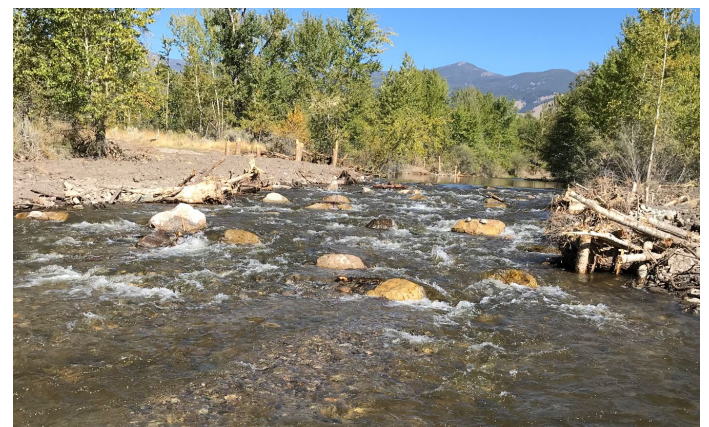
Constructed riffle immediately after construction; Lemhi River, ID
