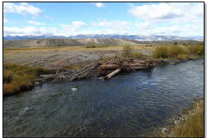
LWM habitat structure immediately after restoration; Lemhi River, ID
