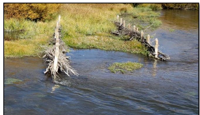
Series of post-line willow-weave bank deflectors creating a point bar; Lemhi River, ID
