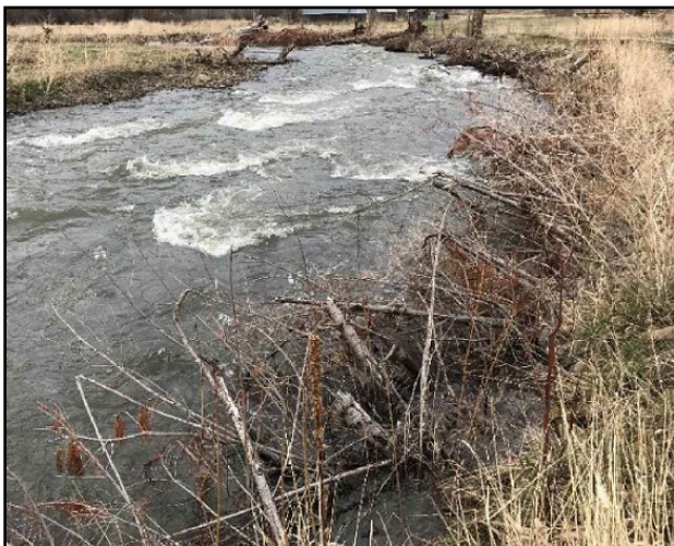
Slash brush layer 1 year after construction; Catherine Creek, OR
