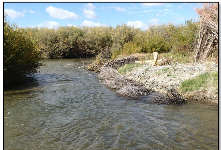
Willow brush layer during construction (Above) and immediately after construction (Below); Lemhi River, ID
