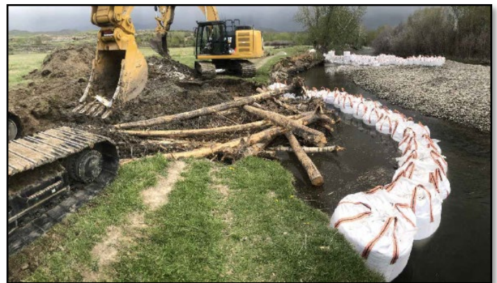
Log bank deflector structure during installation; Lemhi River, ID
