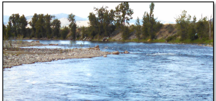
Series of low-profile wood and rock bank deflectors used to narrow the effective channel width and define the thalweg; Methow River, WA
