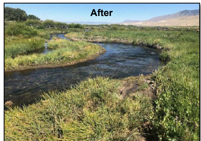
Big Springs Creek 1 year after construction; Width-to-depth ratio reduced by over 50% using FESL on both banks
