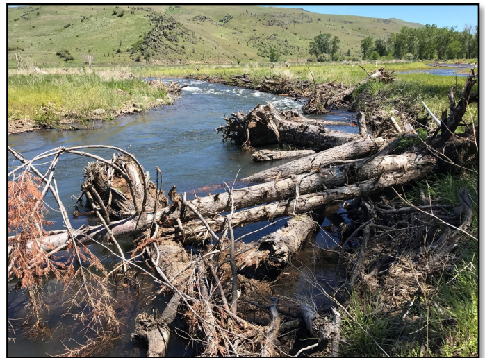
Newly constructed channel with LWM bank structure 1 year after construction; Catherine Creek, OR
