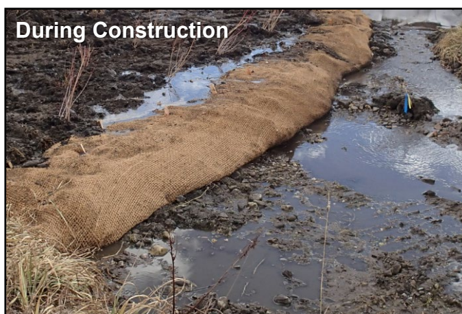
Big Springs Creek during construction; Fill placed behind the FESL with potted plants; Sod mat and potted plants within FESL not yet installed
