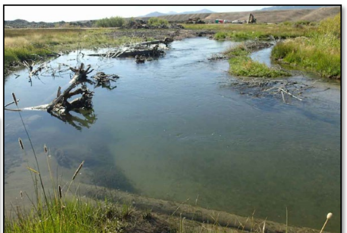
Series of LWM habitat structures 1 year after construction; Lemhi River, ID
