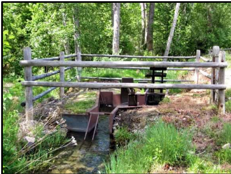
Photo 6. —New NMFS criteria fish screen installed at the Tower Creek -03 (STowC-03) diversion in 2013.
