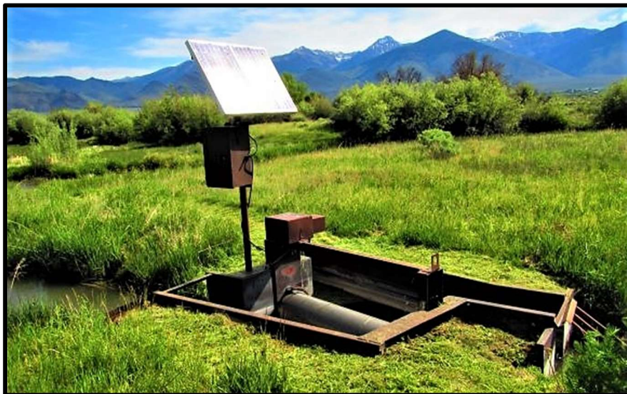
Photo 46. —New NMFS criteria fish screen installed at the Pahsimeroi-10 diversion in 2015.
