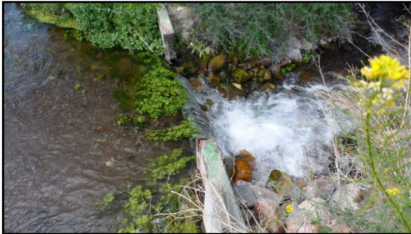
Photo 1. —A previously unscreened diversion on Sulphur Creek dewatered the stream and was a barrier to fish passage.
