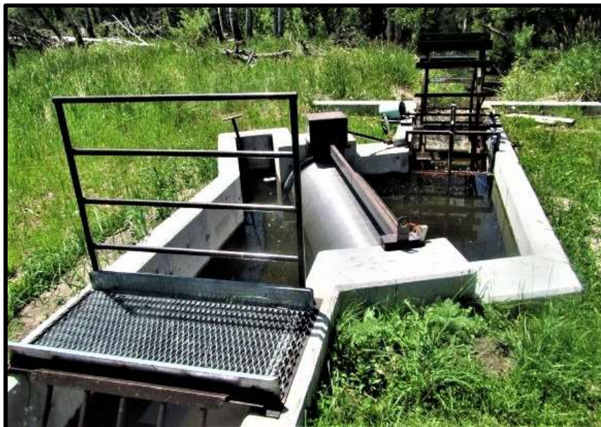
Photo 44. —New NMFS criteria fish screen installed at the Carmen Creek-03 diversion in 2015.
