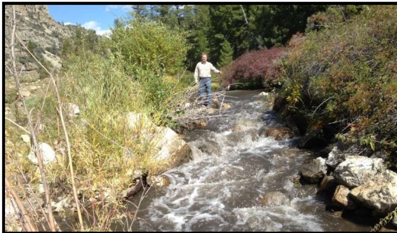
Photo 18. —Old diversion was removed and fish passage was restored on Hawley Creek in 2014.
