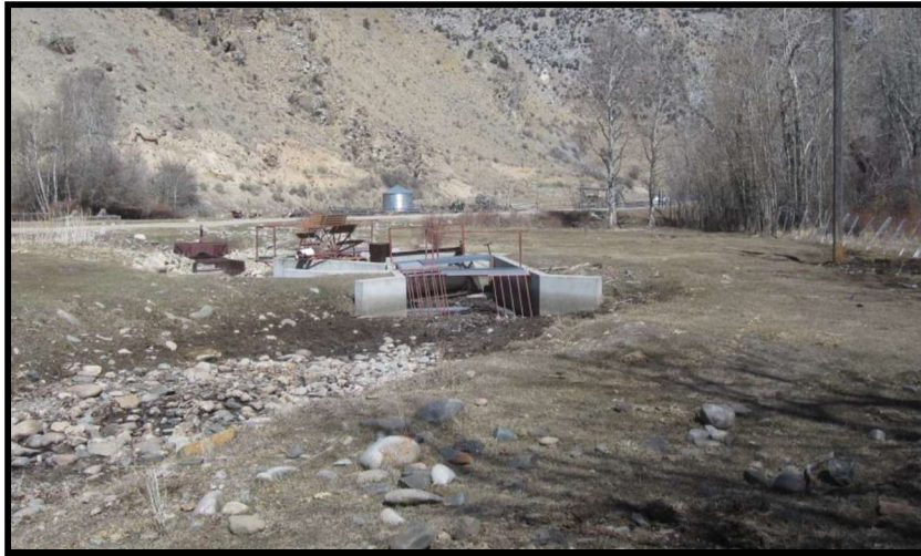
Photo 29. —Old fish screen on the Hayden Creek-08 diversion did not meet NMFS screening criteria.
