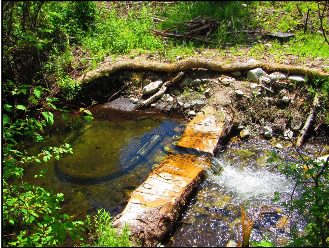
Photo 65. Pratt-Hedt passive fish screen was installed in December 2018. The screen and hose will need to be seasonally removed by the irrigator.
