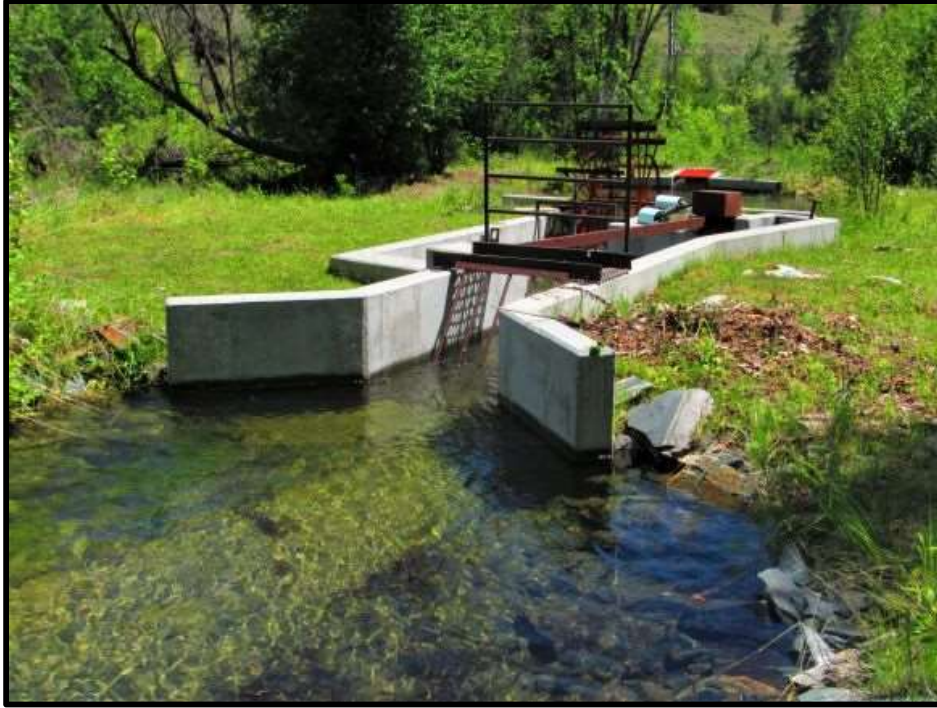
Photo 9. —New NMFS criteria fish screen installed at the Carmen Creek-13 (SCC-13) diversion in 2013.
