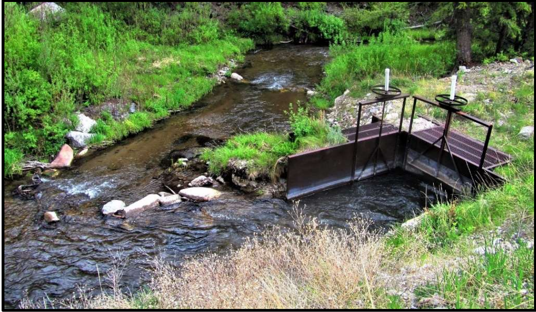
Photo 19. —New diversion and headgate were installed on Hawley Creek in 2014.
