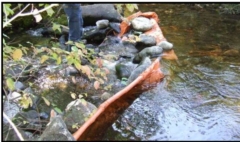
Photo 7. —Previously unscreened diversion on Carmen Creek.
