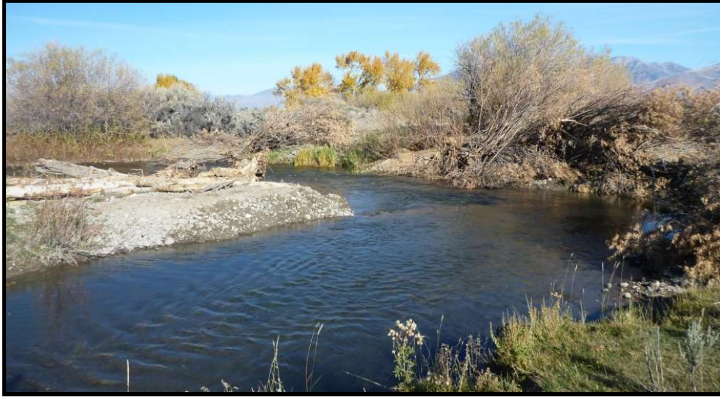
Photo 37. —The site of the old P-16 diversion was rehabilitated and the new diversion allows for fish passage.
