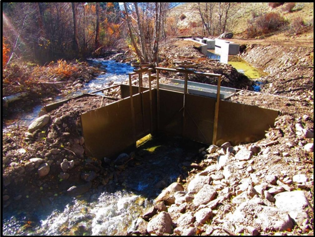
Photo 74. Pratt Creek-03 headgate immediately after installation.
