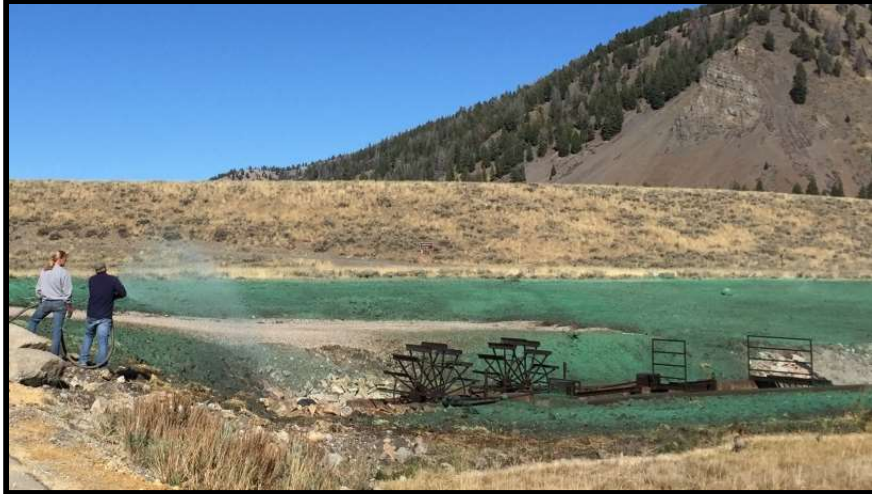
Photo 34. —New NMFS criteria fish screen was installed at the Pole Creek diversion in 2015.
