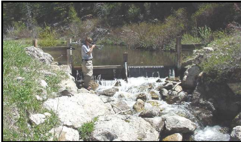
Photo 17. —Previously unscreened diversion on Hawley Creek (LHawC-03) dewatered the stream and was a barrier to fish passage.
