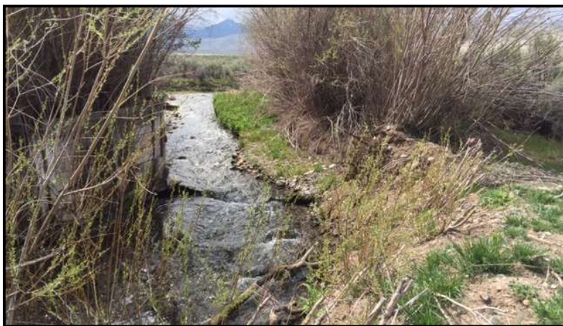
Photo 2. —The old diversion was removed and fish passage was restored on Sulphur Creek in 2014.
