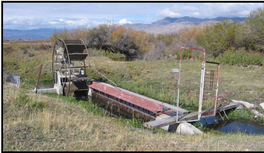
Photo 45. —The old wiper screen on Pahsimeroi-10 diversion before replacement.
