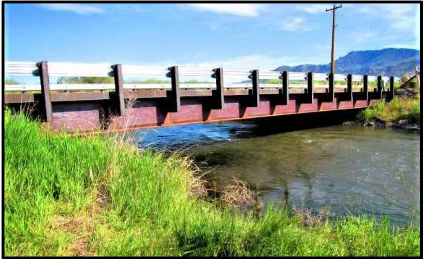
Photo 53. —New bridge across the Pahsimeroi River at Dowton Lane was installed in 2016 to eliminate a passage barrier.
