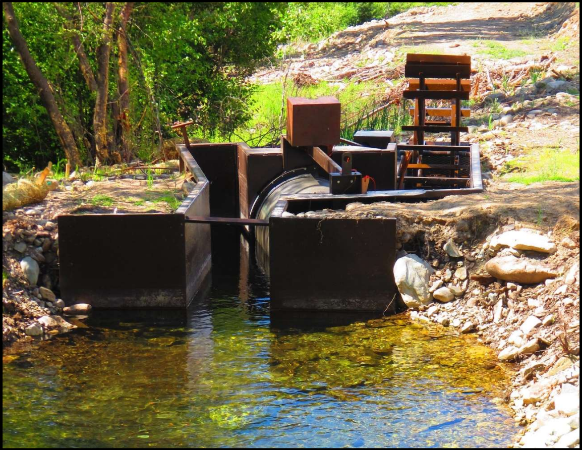
Photo 72. Pratt Creek-02 (LPrC-02) fish screen was installed in spring of 2019.
