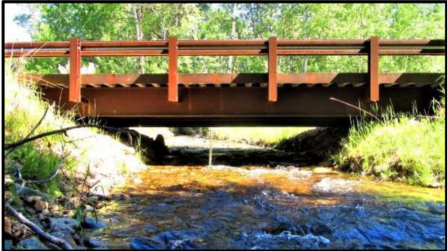
Photo 49. —New bridge across Bohannon Creek was installed in 2015 to eliminate a passage barrier.
