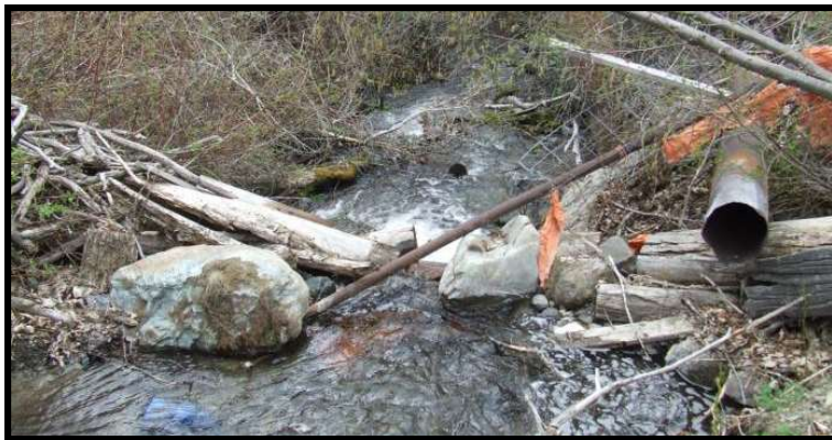
Photo 27. —Previously unscreened diversions on Poison Creek (SPoiC-1) dewatered the stream and were barriers to fish passage.
