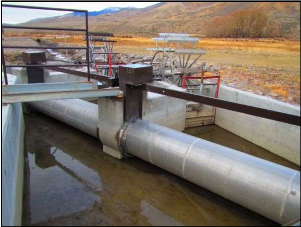
Photo 64. A new NMFS Criteria fish screen is replacing a fish screen that was not functioning properly due to age and poor drainage. The concrete was poured and screen fabricated in 2018, but the screen will not be completed until the headgate and ditch works were installed in spring of 2019.
