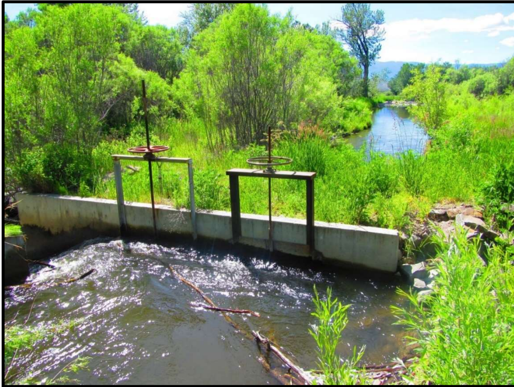
Photo 69. The L-08A ditch was enlarged to accommodate the additional water.
