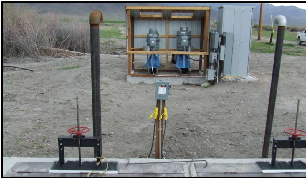
Photo 26. —The new Pahsimeroi-13 pump station allows for the reconnection of Sulphur Creek to the Pahsimeroi and maintains flow and fish passage in the Pahsimeroi River in this reach.
