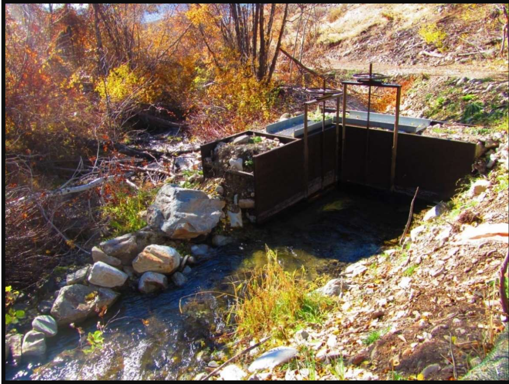
Photo 73. Pratt Creek-02 headgate.
