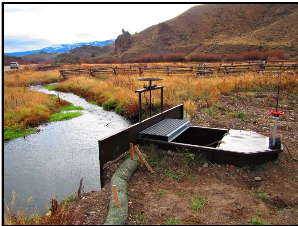
Photo 78. A new NMFS Criteria fish screen was installed on Little Sawmill Creek-01.
