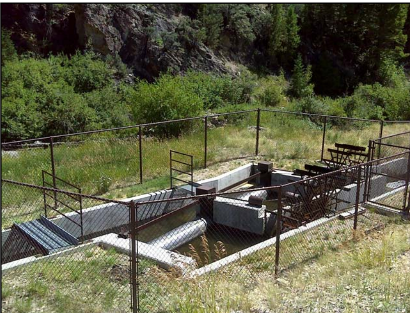
This fish screen was installed on Hawley Creek -03 diversion as part of the cooperative project to reconnect Hawley Creek to the Lemhi River.
