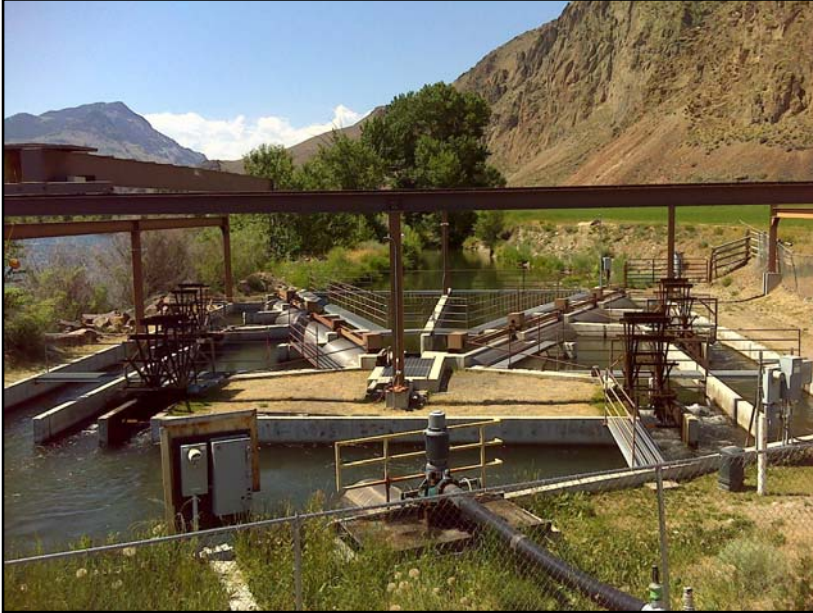
The S-28 diversion fish screen on the Salmon River near Challis is one of the largest screens in the program.
