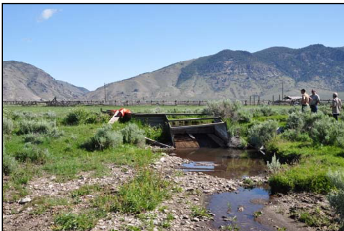
Unscreened diversion on Hawley Creek prior to removal, June 2015.
