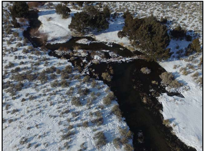
Looking downstream at one of the structures installed in winter 2017.
