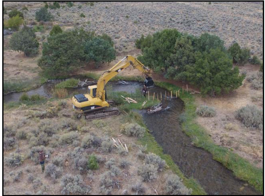
The desirable method for installing the posts is a handheld hydraulic post pounder, however when that didn't work we improvised; spring 2017.
