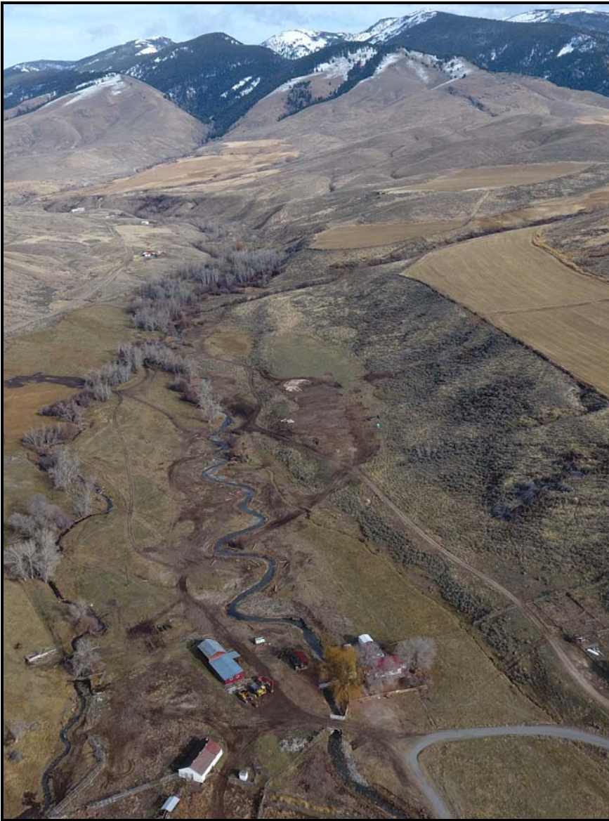
Wimpey Creek project site after instream work was completed, November 2017. Photo by Lost River Fish Ecology.
