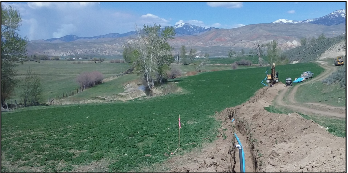
Pipe installation on the Carmen Creek Flow Enhancement Project, April 2015
