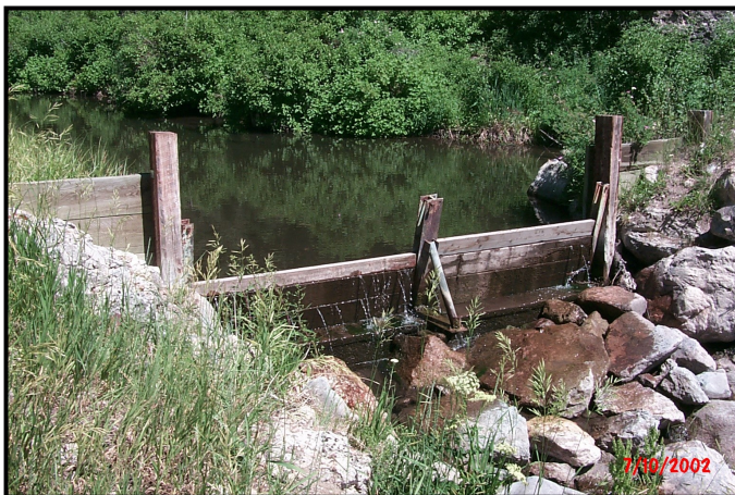
The unscreened diversion on Upper Hawley Creek prior to removal, July 2002
