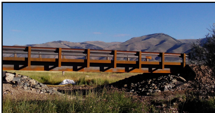
The new Eighteenmile Creek Bridge, Aug. 2015
