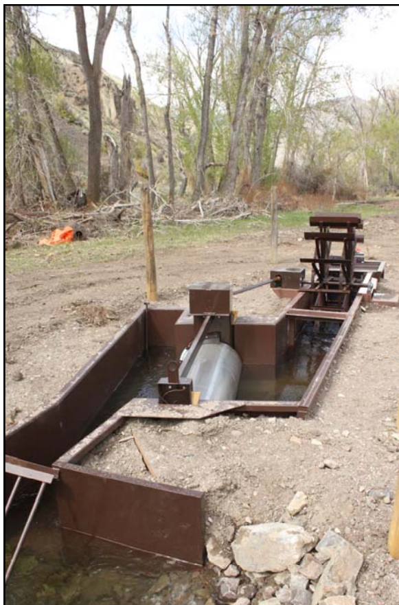
Installation of the new fish screen.
