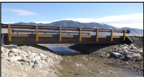
The Hawley Creek culvert (top photo) was replaced with a new fish-friendly bridge (bottom photo).
