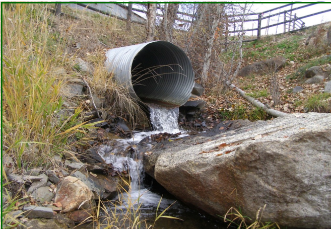
The Wallace Creek culvert is impassable to fish seeking out cold water refugia.
