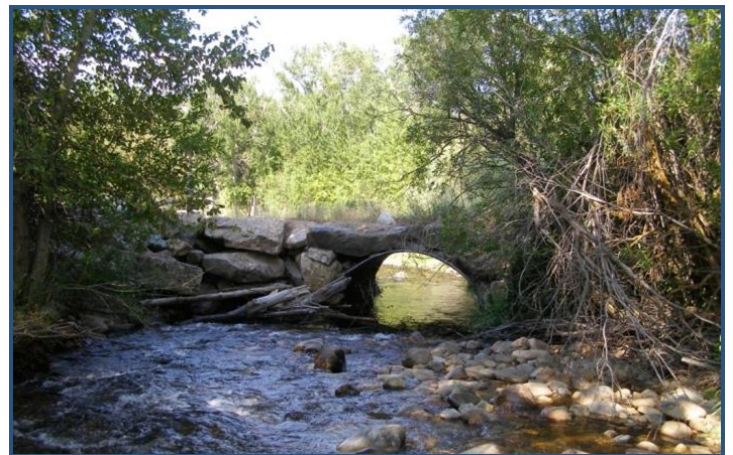
The left culvert on Parmenter Lane on Carmen Creek blocked by debris.
